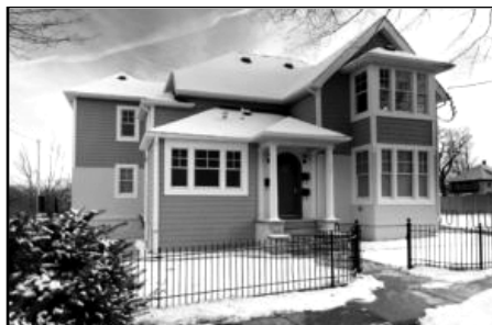
"After" on Eddy Street in Flint (Photo provided by Land Bank)
