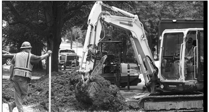
Flint water pipe replacement crew (Photo by Edwin D. Custer)
