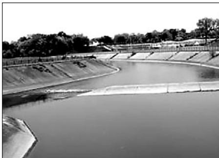
Flint River-Swartz Creek Confluence: Flint River front/right meets Swartz Creek on the left; Atwood Stadium in the background; view from the south. Photo by HC Ford
