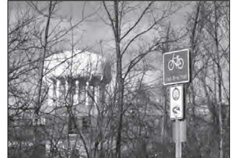
Flint water tower on north Dort Hwy. (Photo by Tom Travis)
