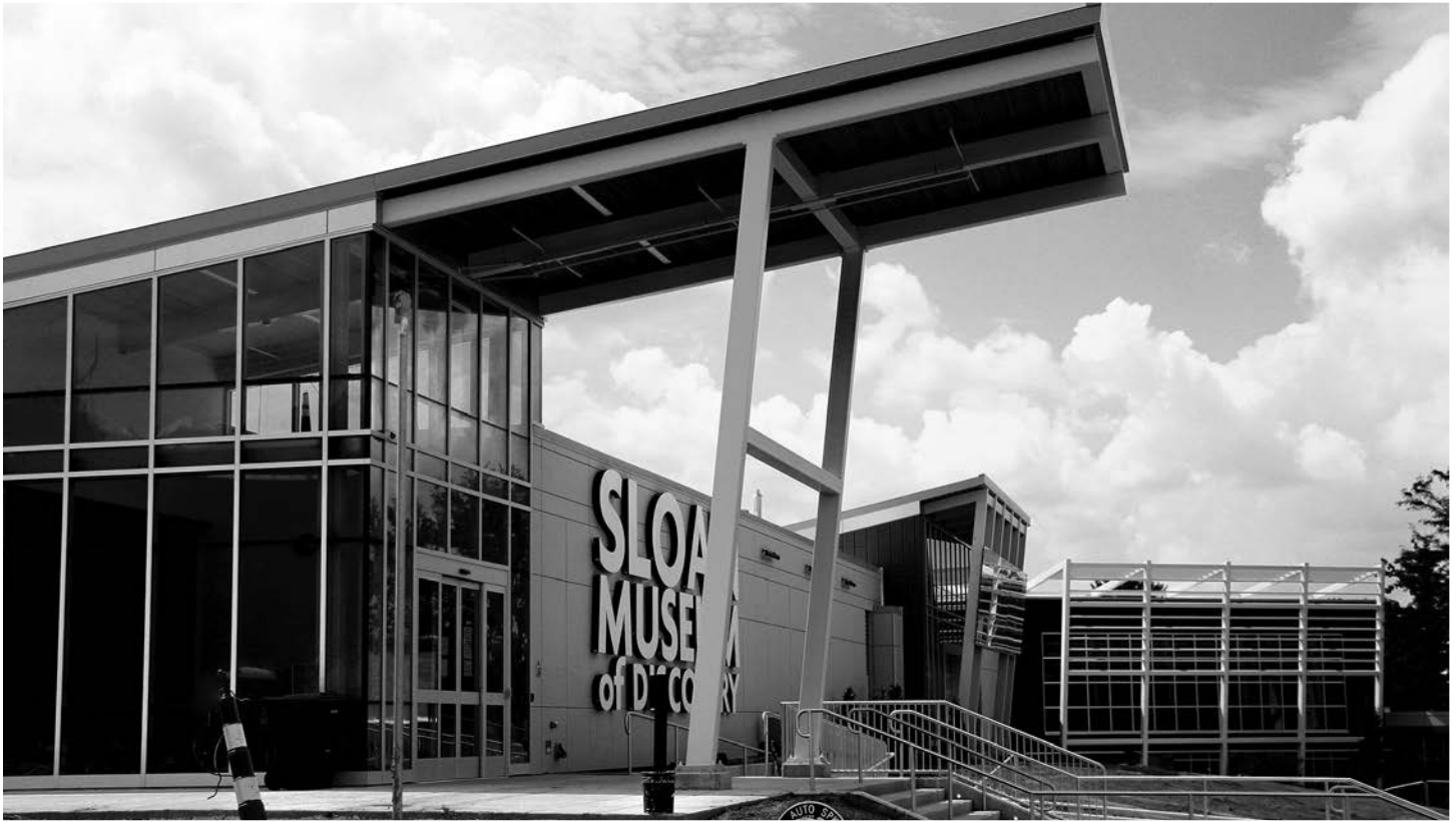
Photo of the Month: Cultural Center as work continues
