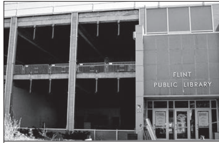
The Flint Public Library during renovations in 2020-21
