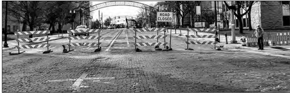
Construction begins on Saginaw Street downtown Flint in April 2023
