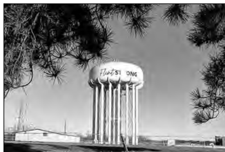
Flint Water Tower
